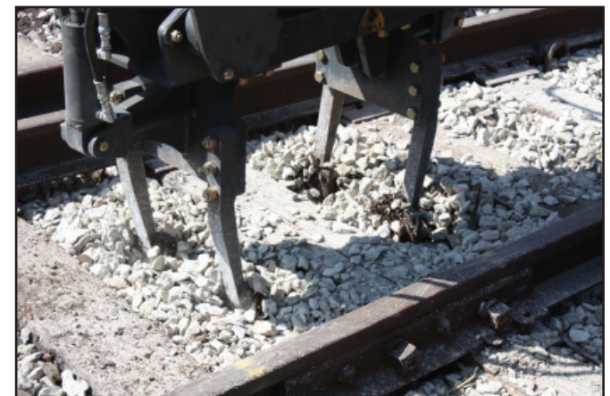
While vibrating in the ballast use the tool squeeze cylinders to force ballast beneath the tie.
