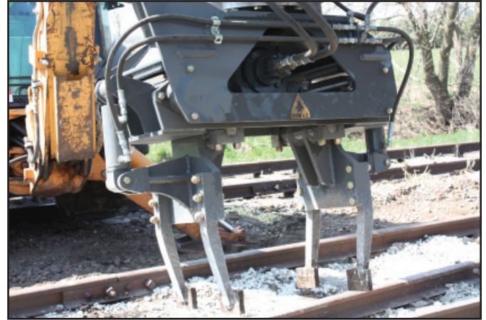
Initial engagement of Dymax DBT.1 plunging into ballast.
