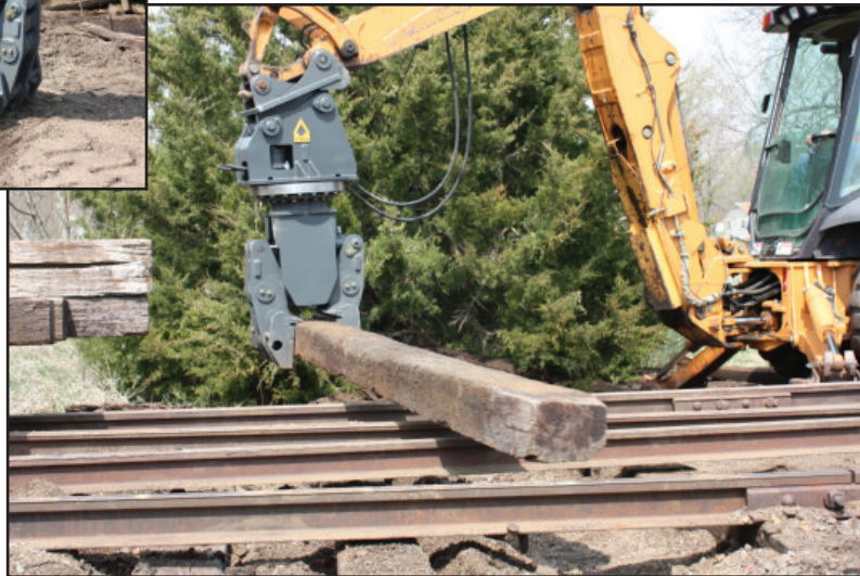
Shown handling wood switch ties.
